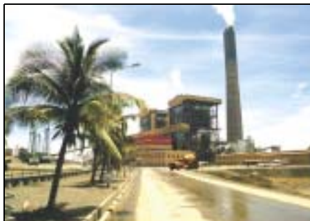
Fig. 9 One of SRL’s recent projects – a power plant in the Philippines
